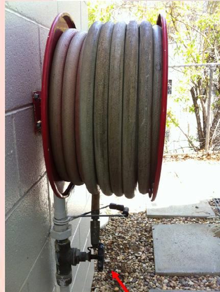
Hose must be inserted through the hose guide and secured in the nozzle lock. Pressure must also be released from the hose and then the hose nozzle turned to the off position.
